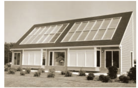
Built at UD with support from Delmarva Power and Light Co., and dedicated in 1973, SOLAR ONE was the first experimental house to directly convert sunlight into both heat and electricity for domestic use.
